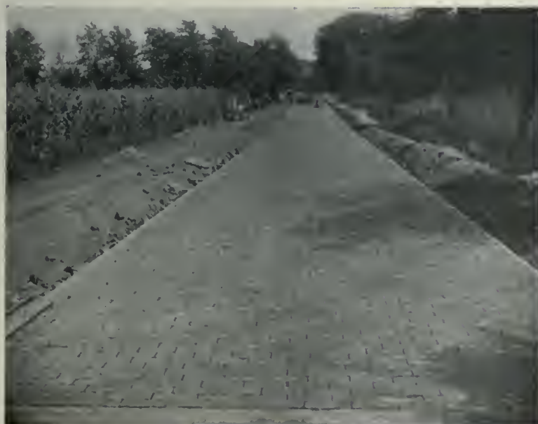
Fig. 2—Completed brick pavement, Paris, Ill.
